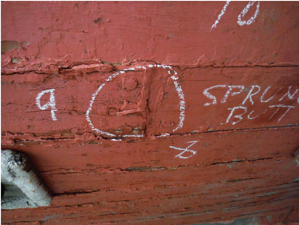
SPRUNG & POOR BUTT
