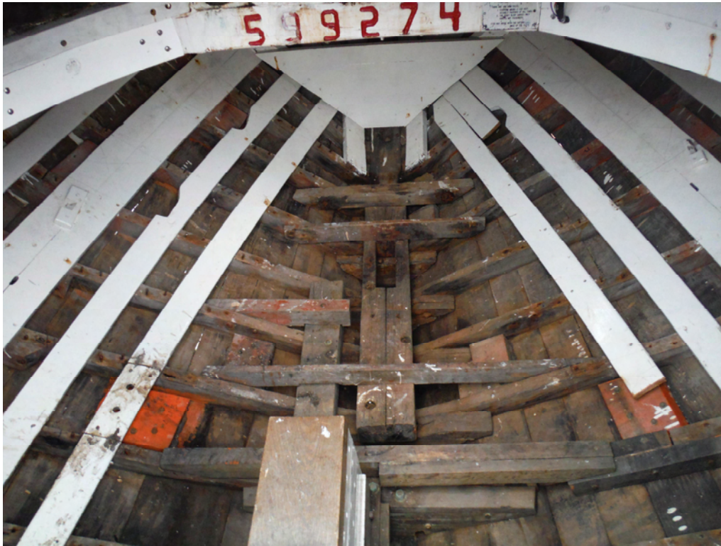
LOOKING FORWARD IN THE CABIN
